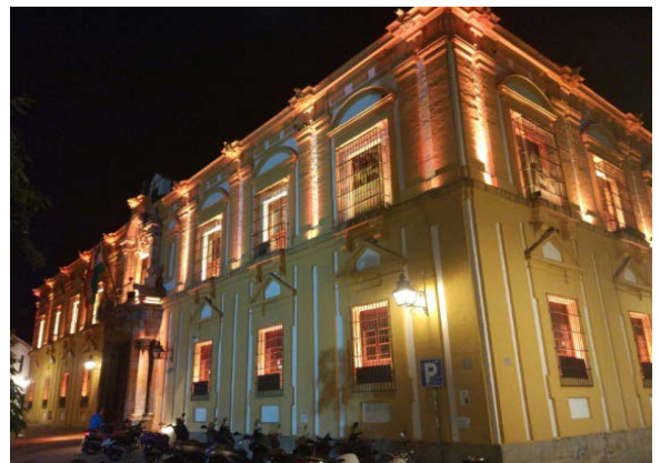
Figure 3. General view of the building object of the competition with the luminaires used.
