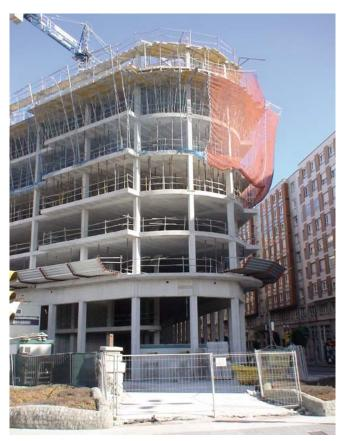
Figure 9. Rotated pillars of the façade perimeter.
